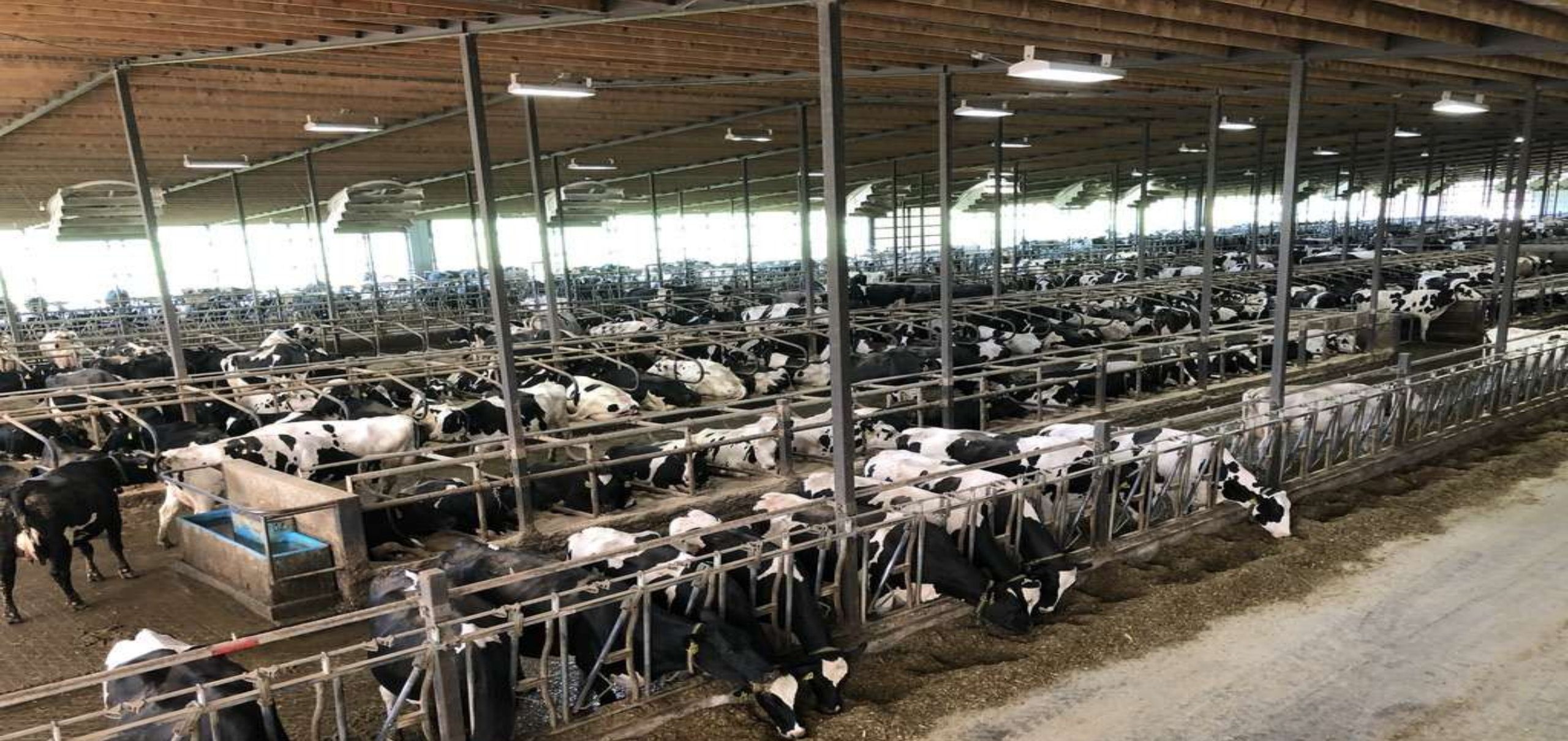
Cross-Vents without baffles use fans to create the air speed in the stalls
